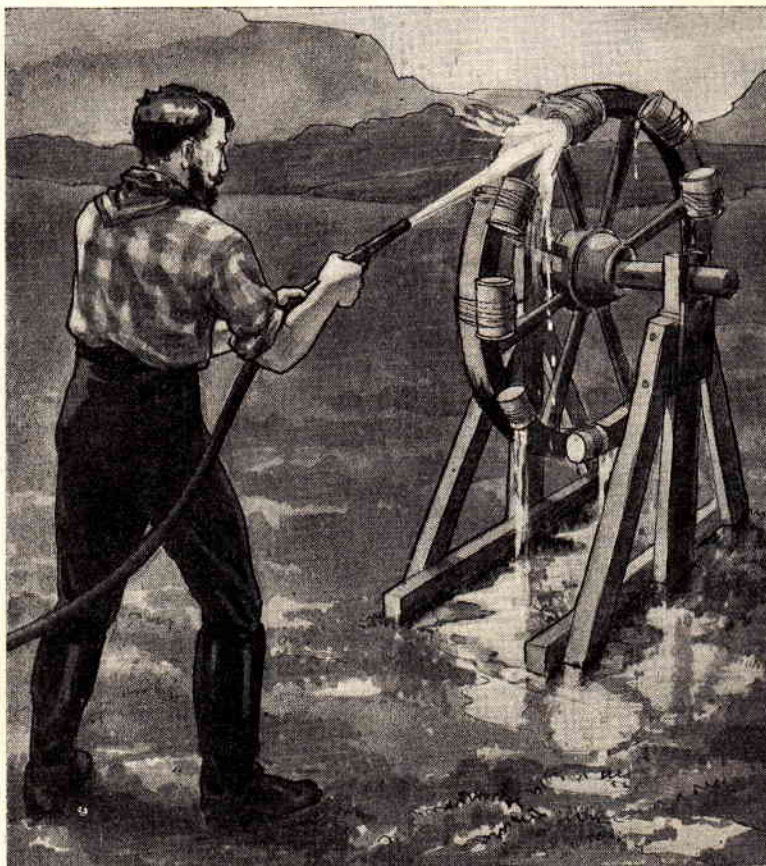
The very first Pelton Wheel made by tying old cans to a waggon wheel
